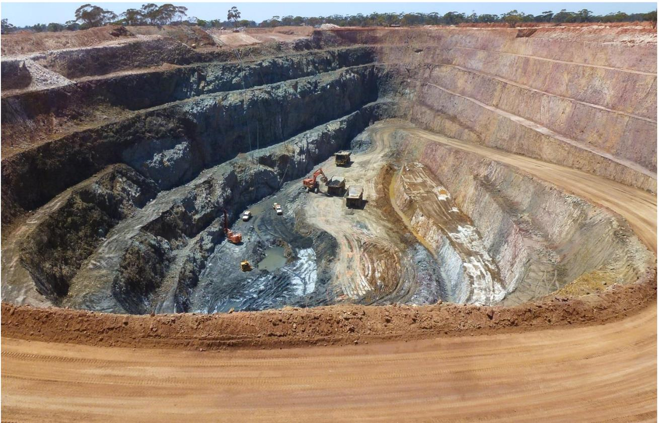
**Figure 1 : Penny's Find Open Pit looking south. Free dig, deeply weathered footwall sediments are to the right, fresh competent hanging wall basalts requiring drill and blast are to the left. The proposed underground portal would be located just below the excavator in the photograph.**
