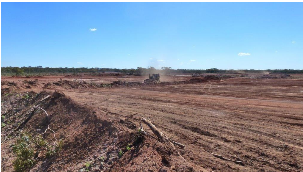
Clearing top soil over pit area ready for transport and storage
